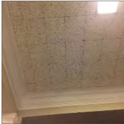
Asbestos-containing 12" x 12" glued-on ceiling tiles, scattered dot and fissure pattern, Storage Room adjacent to Margaret Charter's Auditorium, Level 1 McMaster Wing.
