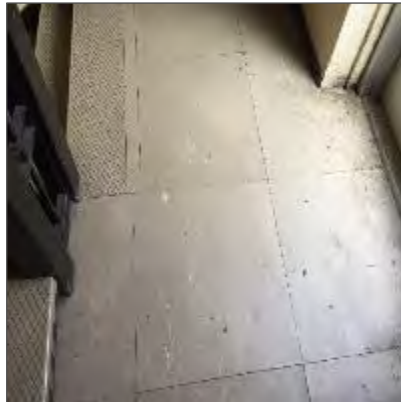
Non-asbestos brown vinyl flooring, Stairwell to Basement.
