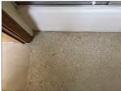
Photo 3 – Non-asbestos vinyl sheet flooring, beige pebble pattern, Level 1 South-west Former Washroom.
