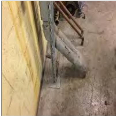
Asbestos-containing paring cement on pipe fittings, East Wing Mechanical Penthouse.
