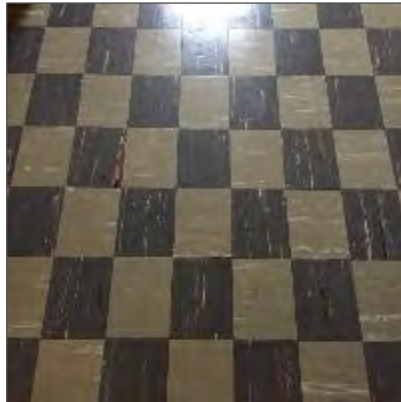
Photo 1 – Asbestos-containing 9" x 9" vinyl floor tile, green/grey in checker pattern, Second Floor Intern's Room.
