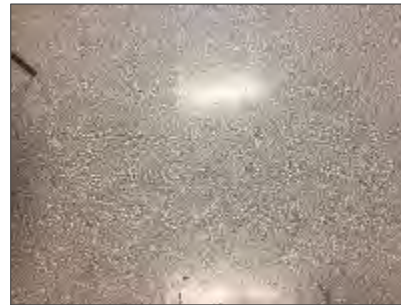
Photo 4 – Non-asbestos vinyl sheet flooring, dark grey pebble pattern, Level 1 Kitchen Area.
