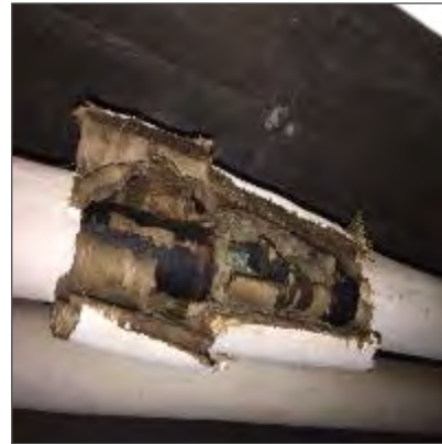
Suspect asbestos-containing Sweatwrap on pipe straight, Basement.
