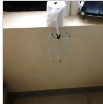
Photo 2 – Damaged asbestos-containing plaster on wall, Intern's Residence, Level 2 Washroom adjacent to Main Stairwell.
