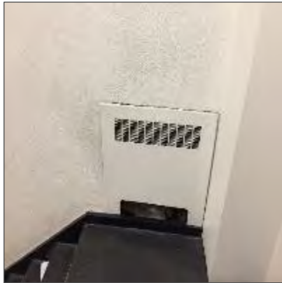
Photo 7 – Asbestos-containing plaster debris below radiator, Landing between Level 1 and 2, South Stairwell of McMaster Wing.
