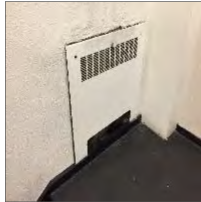
Photo 8 – Asbestos-containing plaster debris below radiator, Landing between Level 2 and 3, South Stairwell of McMaster Wing.
