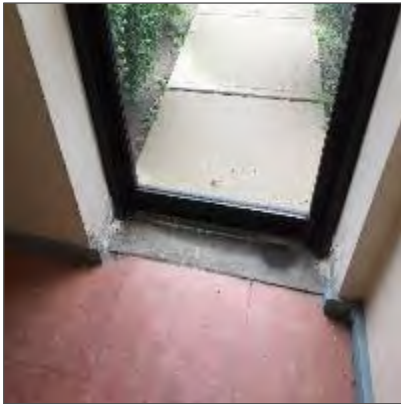
Photo 1 - Damaged asbestos-containing plaster and debris at exit door, Intern's Residence, Main Stairwell.
