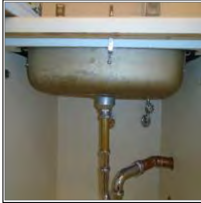
Asbestos-containing metallic undercoating on the bottom of a sink, Level 2 Operating Area.
